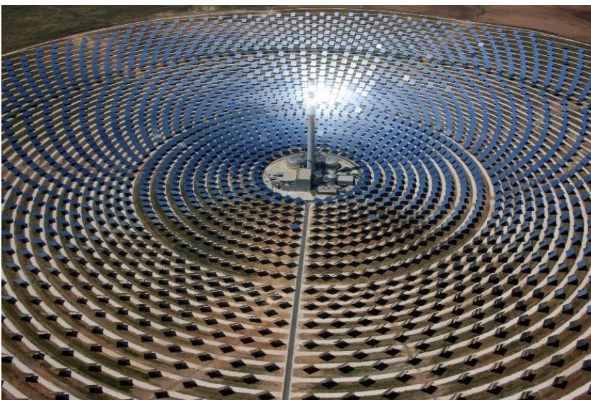
Note: aerial view of the Gemasolar plant in Spain, Source: Castalia, Report to the World Bank, 2020, CSP Technology Review and Preliminary Assessment
